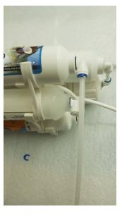
Insert tubing with pulldown adapter. Push tubing inside inside fitting for 1/4", than try to pull tubing out. If tubing insert correctly, tubing stays inside fitting. Insert blue c-ring after (not before).
