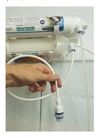
Waste and pure water line have call tags (semiclear tubing is pure water, and white tubing is waste water line)
